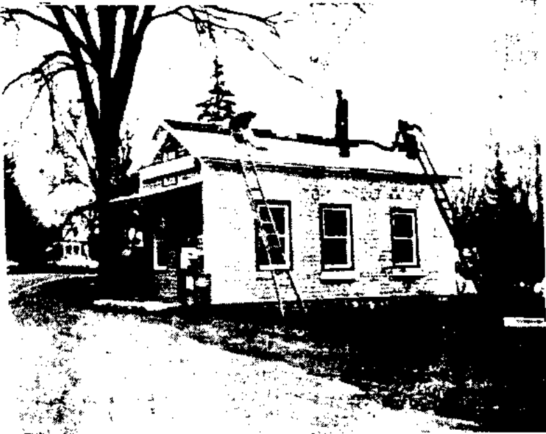
Post Office Roof Project
